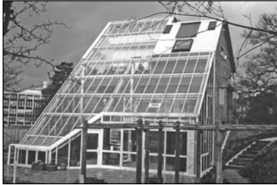
Fig 47 Integer House, near Watford, designed by Cole Thompson, explores new sustainable glass technologies.
